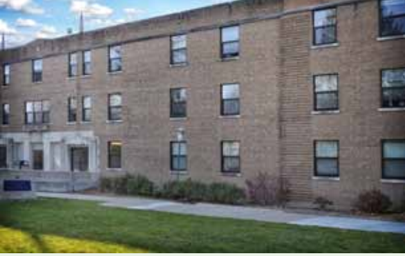
This example shows Lamson Hall retrofitted with a securable archway to access the northern courtyard.
